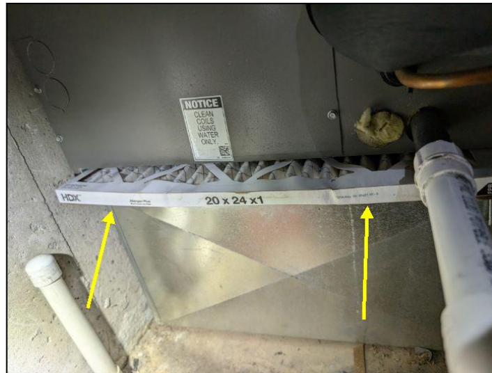
The filter is located here. Size: 20"x24"x1"
